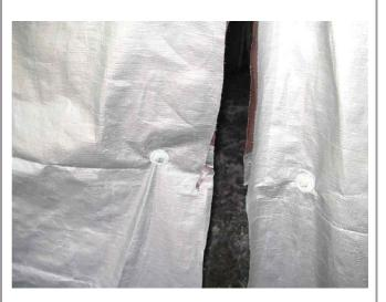
Here is how I held up the middle of the tarp. Two 1/4-20 bolts, one going through a grommet on the tarp edge and the other just punched through the tarp edge.
