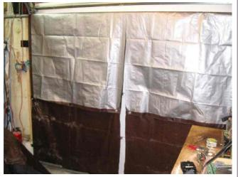
Here is the finished garage door tarp. One interesting thing is that it was not folded squarely. Measure the two sides. don't go by the folds in the material. You can see the center split has opened up a bit. I might move the bolts down a bit in the center, but right now I want to keep the split open so I can get the bike tire in the split without pinning a conduit to the floor.
